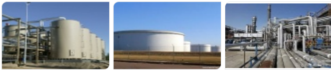
Cleaning Oil Tanks & Pipes
